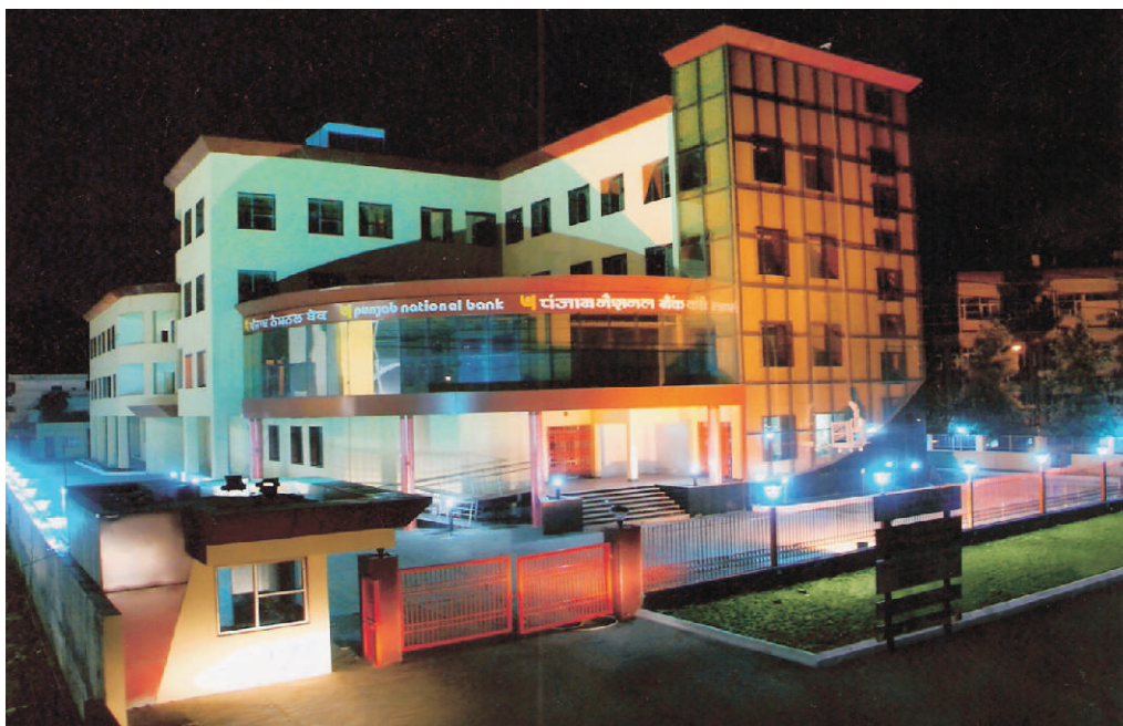
Zonal Office Building for Punjab National Bank, Ludhiana (Punjab)
