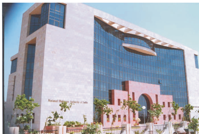
Corporate Office Building of National Highways Authority of India, Delhi
