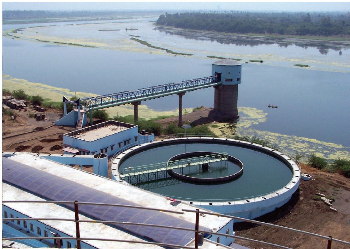
Wss at Variav - View of 10m Dia intake Well in 15m deep riverbed with 14m Dia Pumphouse & 60mld Wtp
